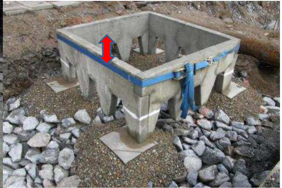
The stone shall fall into the box to get a stable construction
