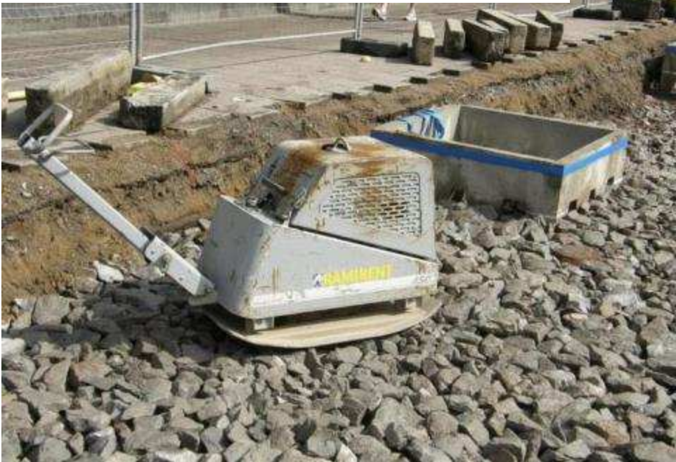
Compacting before soil is washed in to the voids
