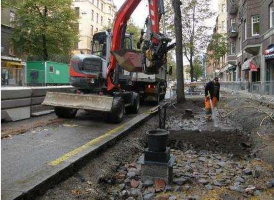
Flushing the soil into the structure
