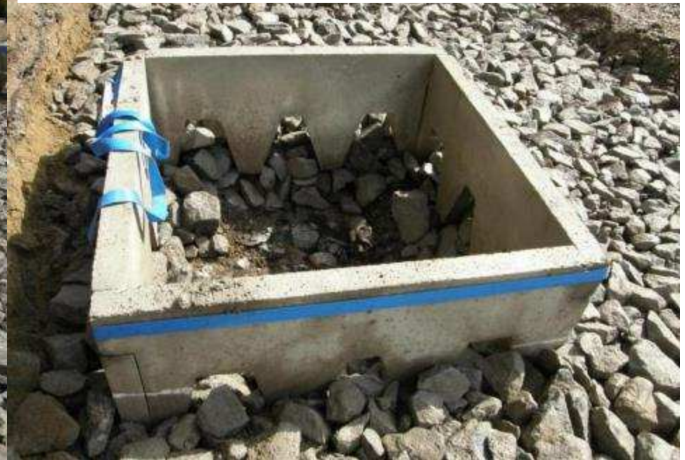
The stone shall fall into the box to get a stable construction
